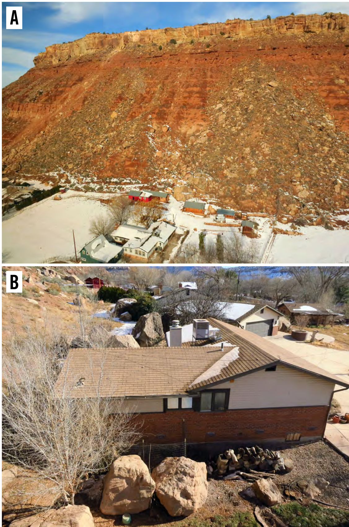
Figure 20. Two views showing structures endangered by rock falls along the base of the Rockville Bench in Rockville, Utah. (A) The white house in the foreground was struck by a rock fall in February 2010. (B) The house in the foreground is immediately east of the December 12 th , 2013, rock-fall site and was struck by small rock-fall fragment; additionally, a very large boulder (figure 16) from that event came to rest only a few feet from this house. Boulders near homes in the middle and far distance are from previous rock falls of unknown timing.
