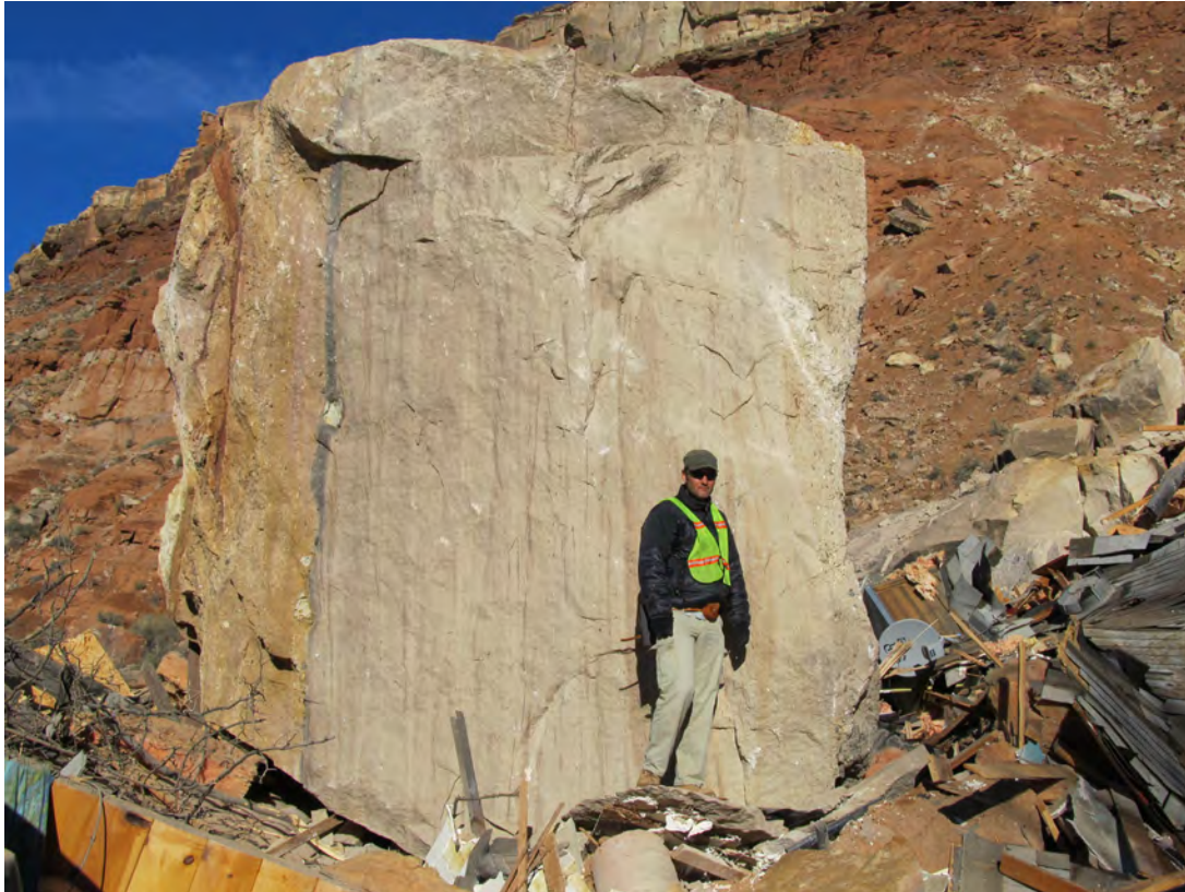
Figure 15. The largest boulder to reach the December 12, 2013, rock-fall site. The boulder is situated within the debris of the destroyed house, and has an estimated volume of 270 yd 3 and mass of 520 tons; average boulder dimensions are 27 x 16 x 16.8 feet. Photograph taken December 17, 2013, view is to the north.
