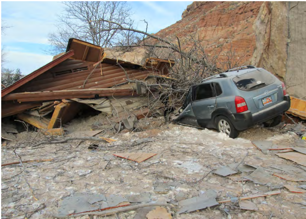
Figure 4. Detached two-car garage and car at 368 West Main Street, Rockville, Utah, destroyed by the December 12, 2013, rock fall. Photograph taken on December 13, 2013, view is to the northwest.
