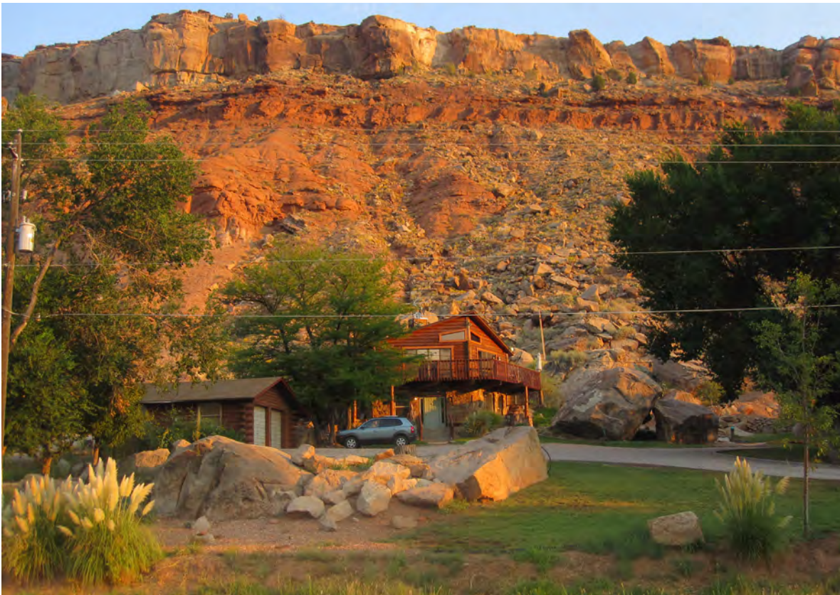
Figure 2. View of the property at 368 West Main Street in Rockville, Utah, taken on September 29, 2010. The house, garage, and car were subsequently destroyed by a rock fall on December 12, 2013; note large pre-existing rock-fall boulders within the property; view is to the north.
